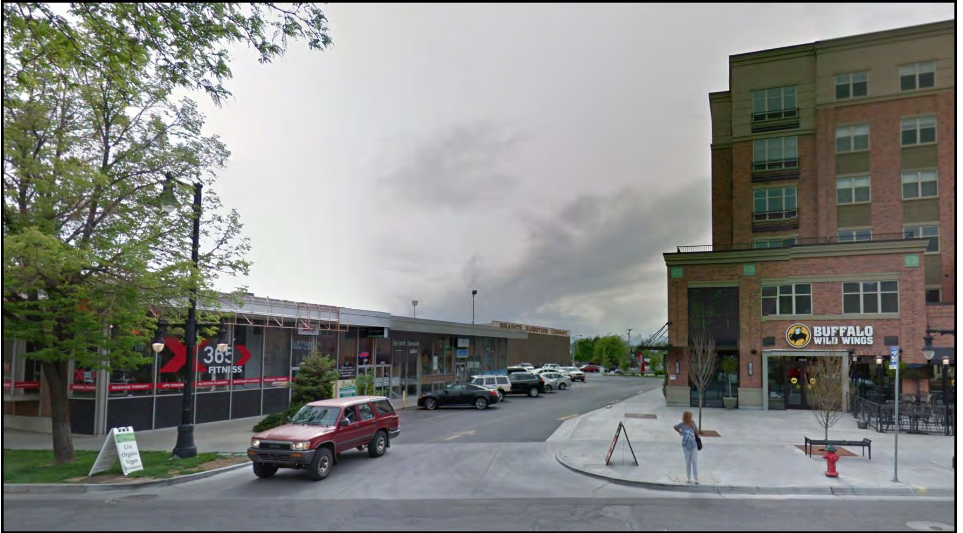
This photograph is looking across Highland Drive towards the southwest. The existing Hyland Plaza slated for demolition is on the left and “The Vue at Sugar House”, a mixed use project also developed by the applicant is on the right. It is proposed that the vehicular access shown in the center of this photograph would be eliminated and replaced with a pedestrian plaza.
